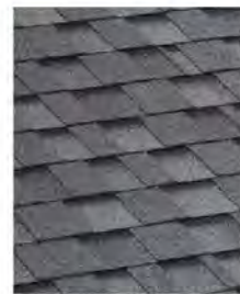
Composition Shingle Roof
