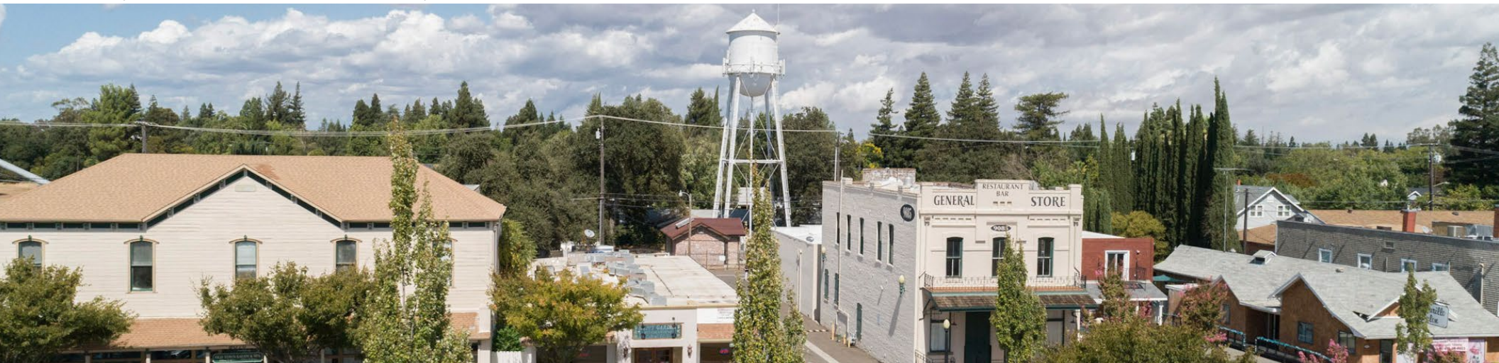
Figure 1. Old Town Elk Grove Along Elk Grove Boulevard
