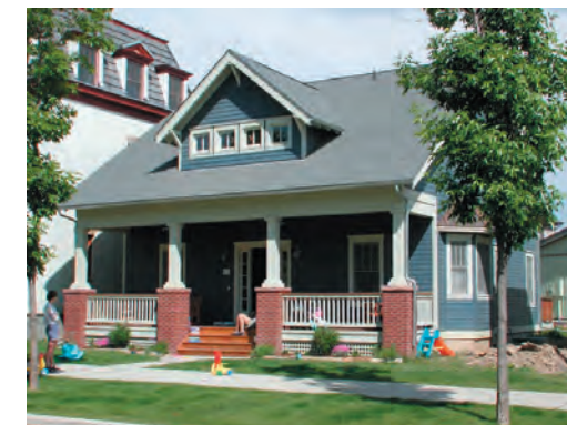
Wide gable dormer
