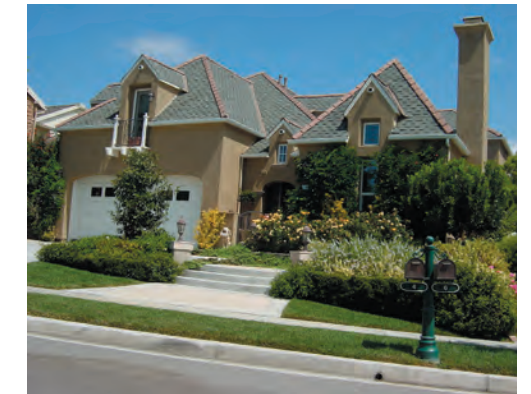
Gable dormers set in hip roof forms
