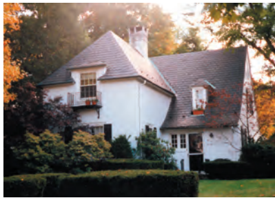
Combination of main roof and dormer roof forms
