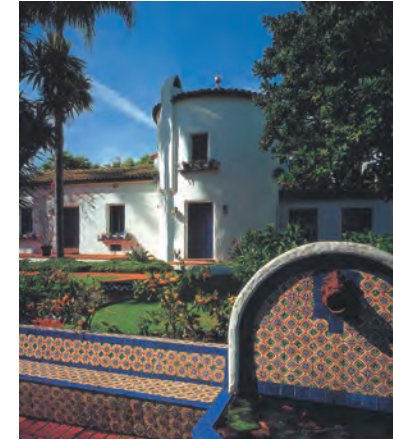
Engaged conical tower
