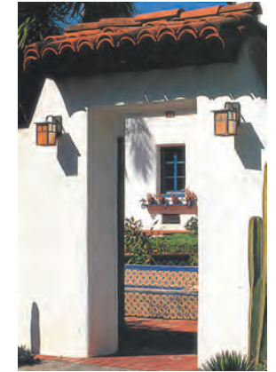
Courtyard entry porticos
