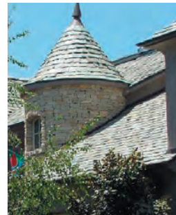
Conical towers with finial
