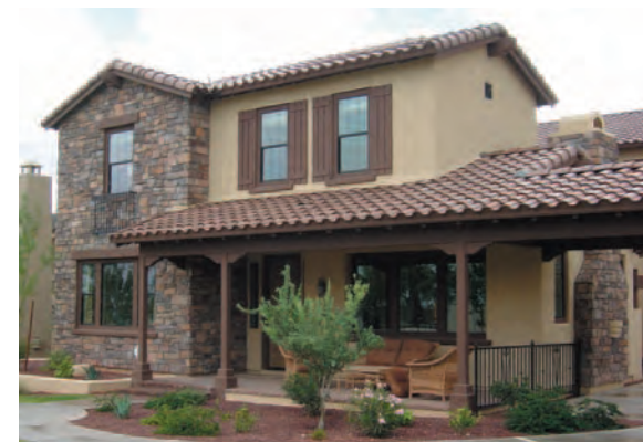
Bracketed porch columns
