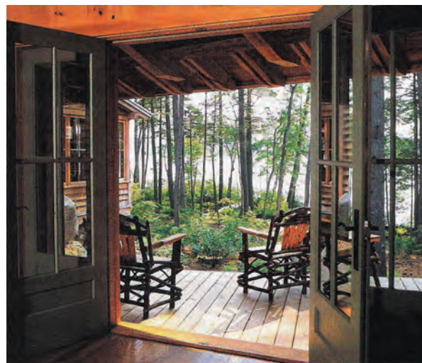
Ganged doors and windows to porch
