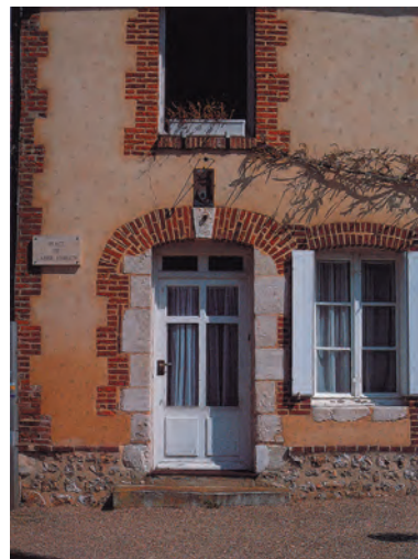
Brick and stone door and window surrounds
