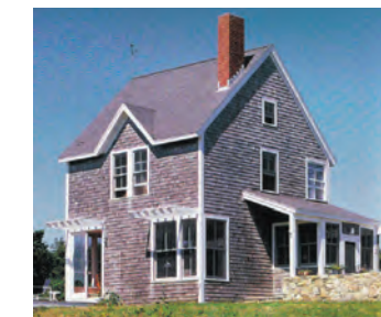
Horizontal siding with corner trim
