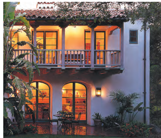
Monterey style balconies
