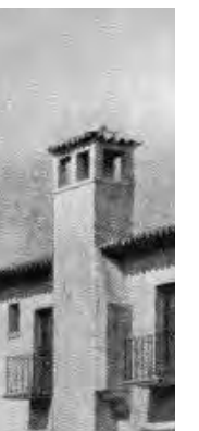
Chimneys with clay tiled hip roofs
