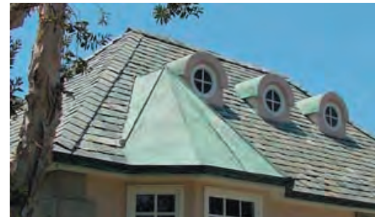
Metal roof material on accent features
