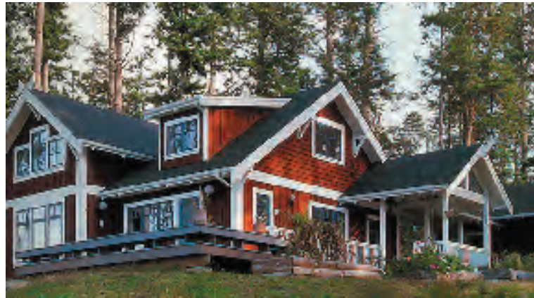
Windows and doors accentuating the elevation
