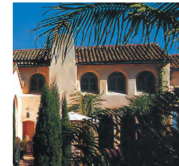
Recessed arched windows
