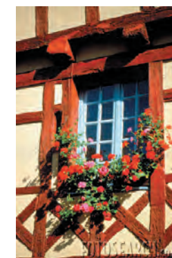
Half timbers in stucco
