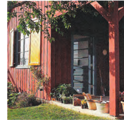
Square posts with angle bracing
