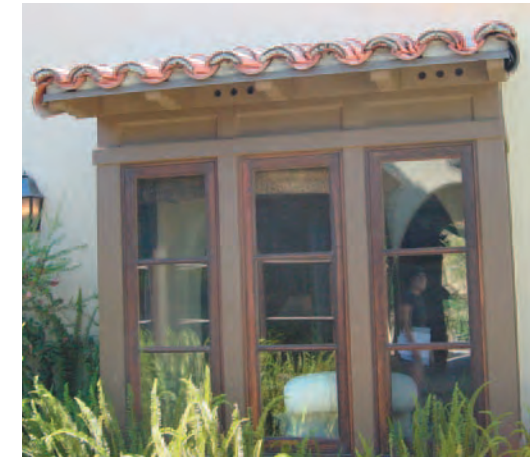
Wood trim window Bay
