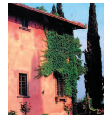
Window grilles were located on the ground floor and either recessed or projected from the wall with carved stone pediments and sills
