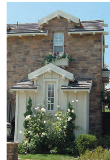
Dormers breaking roof plane
