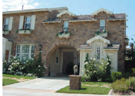
Dormers breaking roof plane
