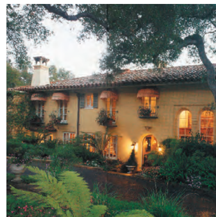
Horizontal 2-story facade villa style
