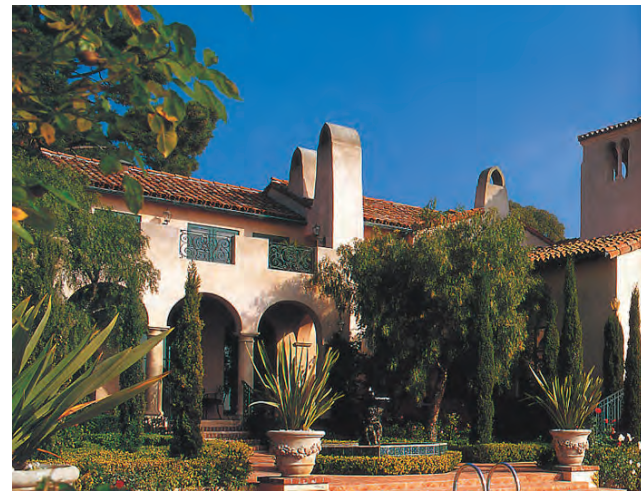
Arched loggia with pre-cast columns
