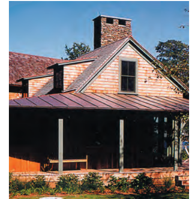
Shed roof dormers
