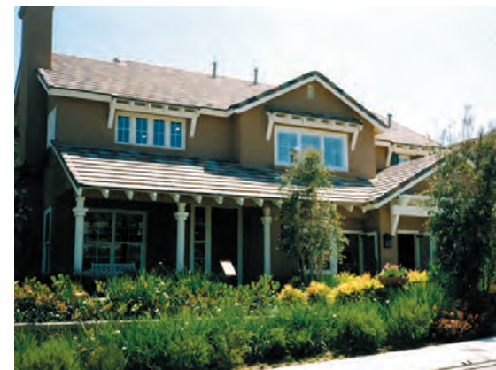
Exposes rafters and timbers
