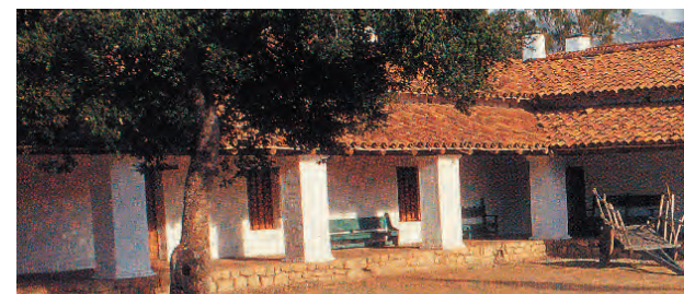
Rectangular loggia columns
