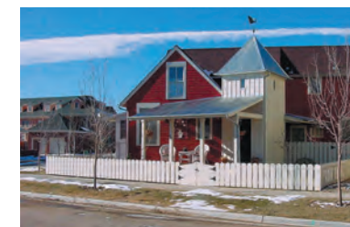
Metal roof accents. Rich colors applied to juxtaposed massing and forms
