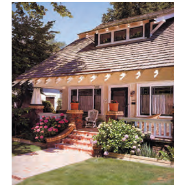
Shed horizontal roof dormer
