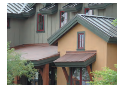
Stucco and board and batten finishes
