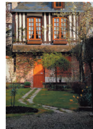
Combination of half-timbers, stucco and brick
