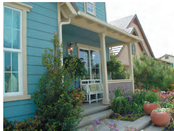
Detailed porch columns and guardrail
