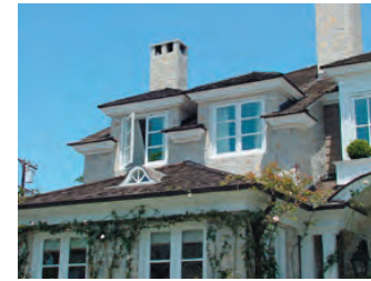
Vertical windows in groupings
