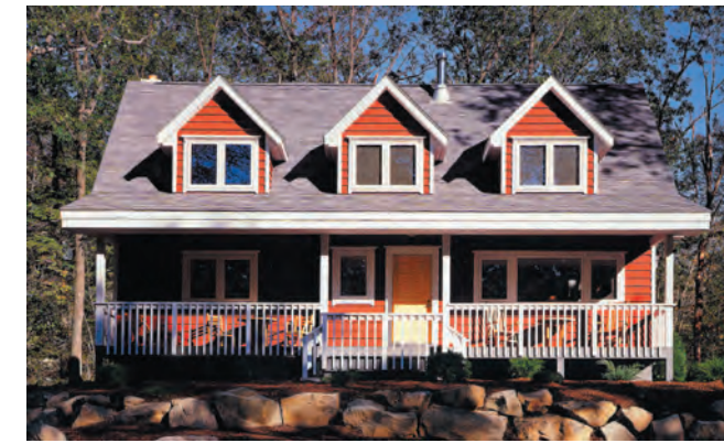
Shallow pitch roof break at porch
