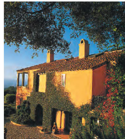
Stucco exterior finish
