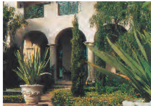
Arched loggia with pre-cast columns
