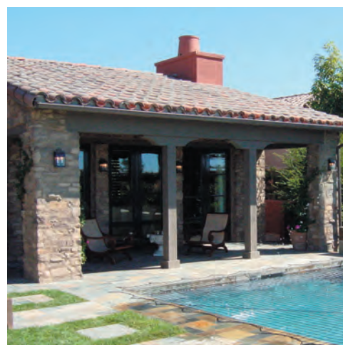
One-story covered loggia
