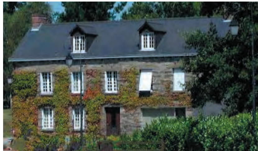
Gable roof dormers
