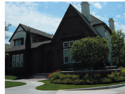
Combination of gable and hip roof forms
