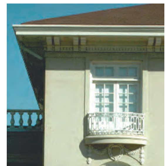
Bracket details at fascia cornice
