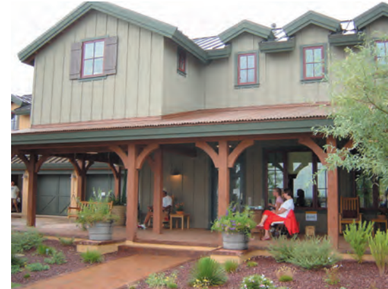
Board and batten vertical siding
