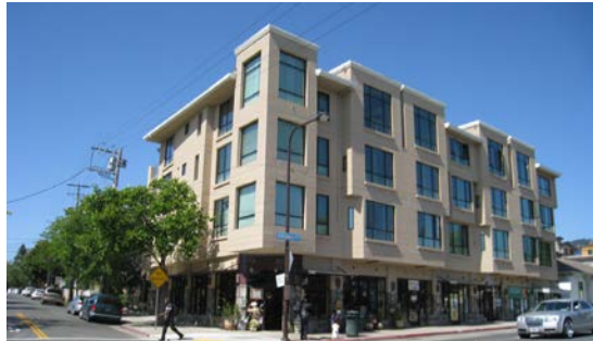
All building sides have glazing, projections and recessed elements
