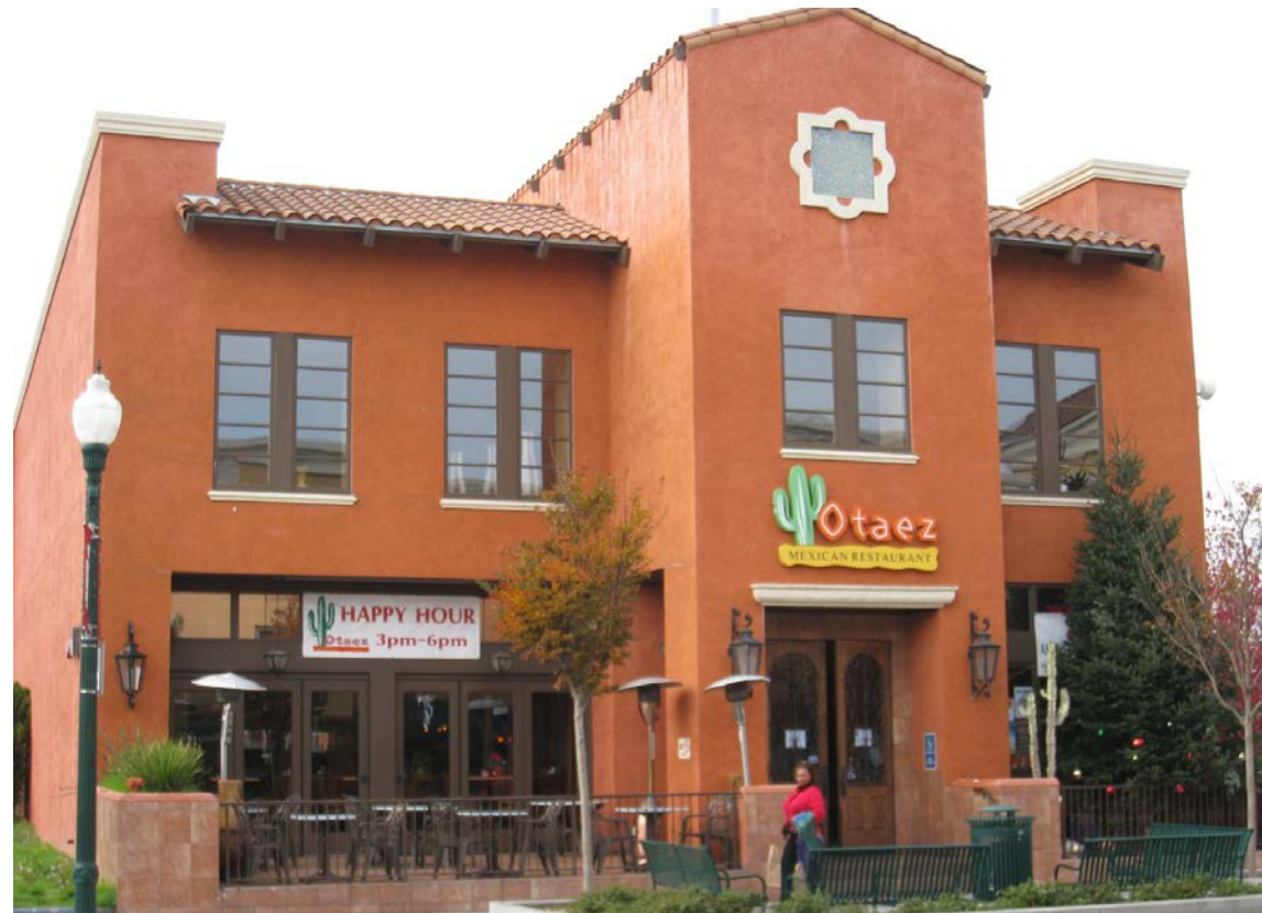
Varying cornices and rooflines
