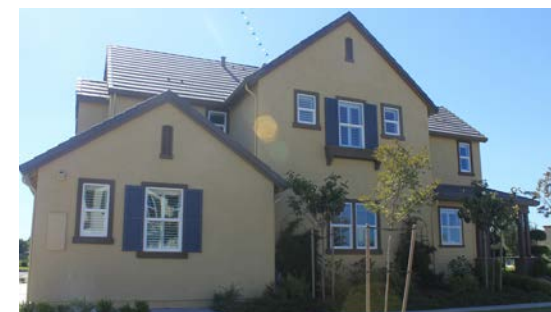
Enhanced window openings
