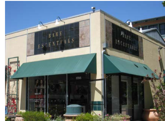
Glazing, lighting and awnings enhance facade
