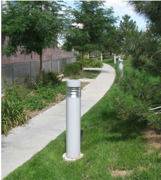
Bollard lighting of pedestrian walkway
