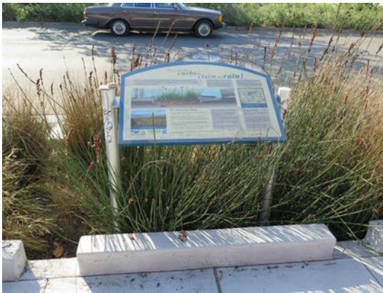
Landscaped stormwater planters
