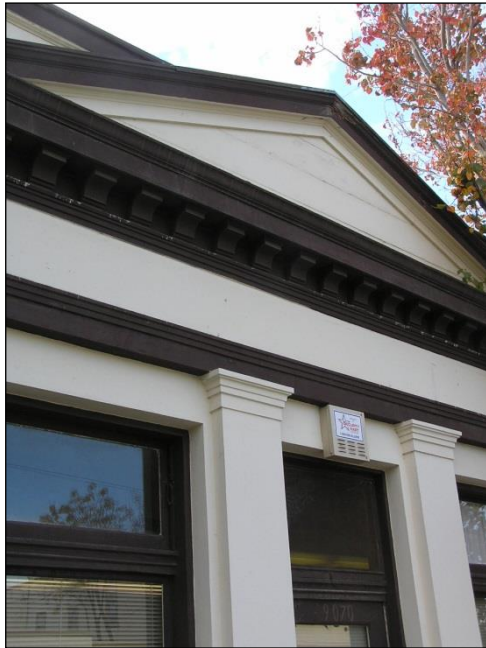
G. 9070 Elk Grove Blvd. (South side of Elk Grove Boulevard)
