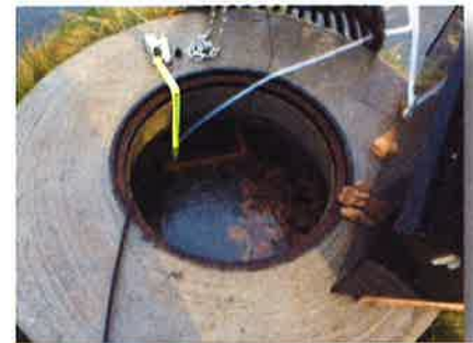
Figure 4. Looking into the sedimentation well at CY, January 5, 2016.
