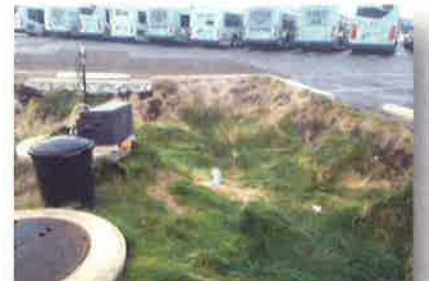
Figure 2. Dry well at CY, November 2, 2015.
