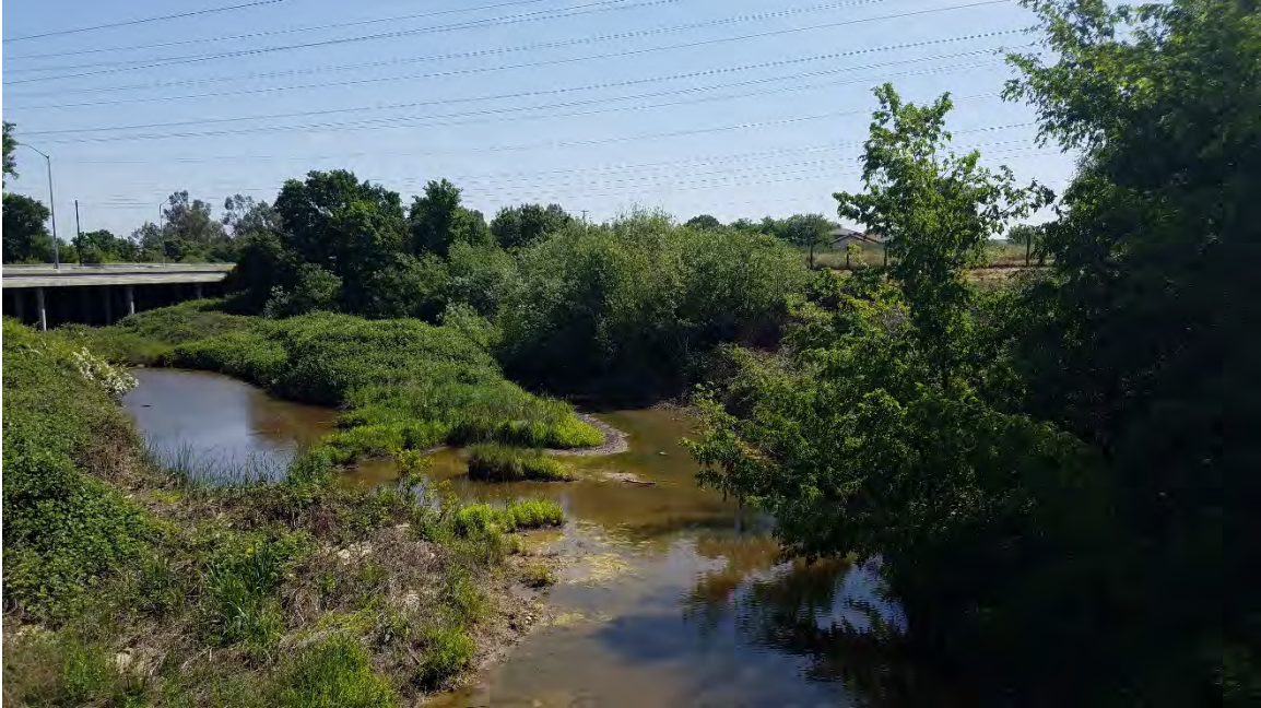
Arterial Roads Project.170242
