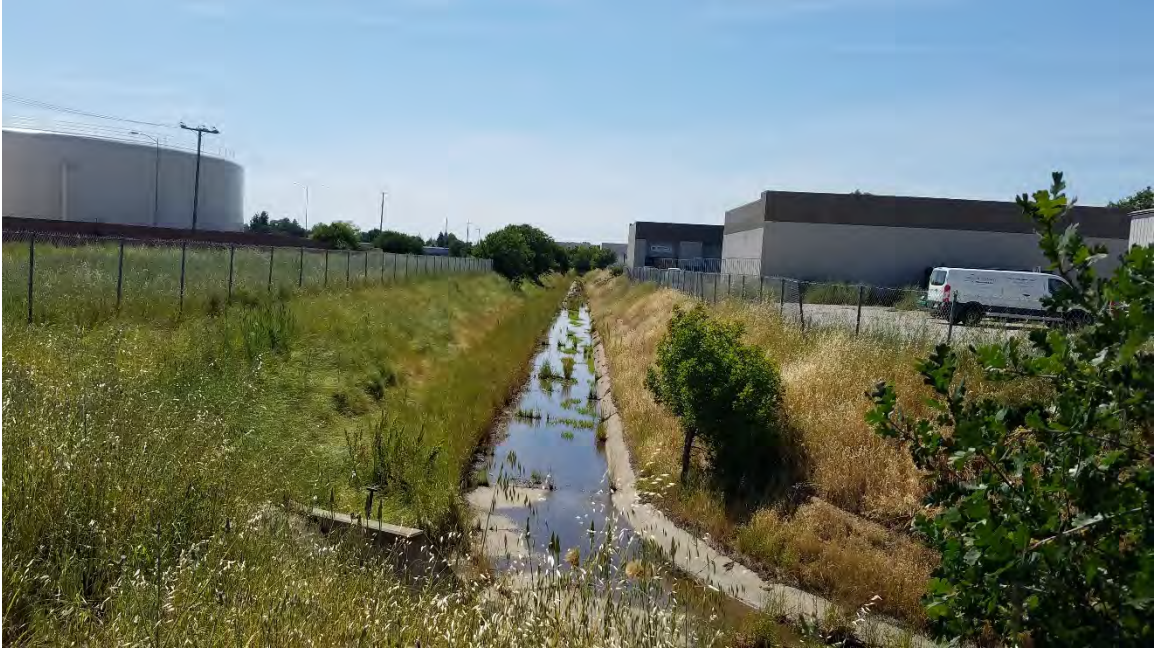
Arterial Roads Project. 170242
