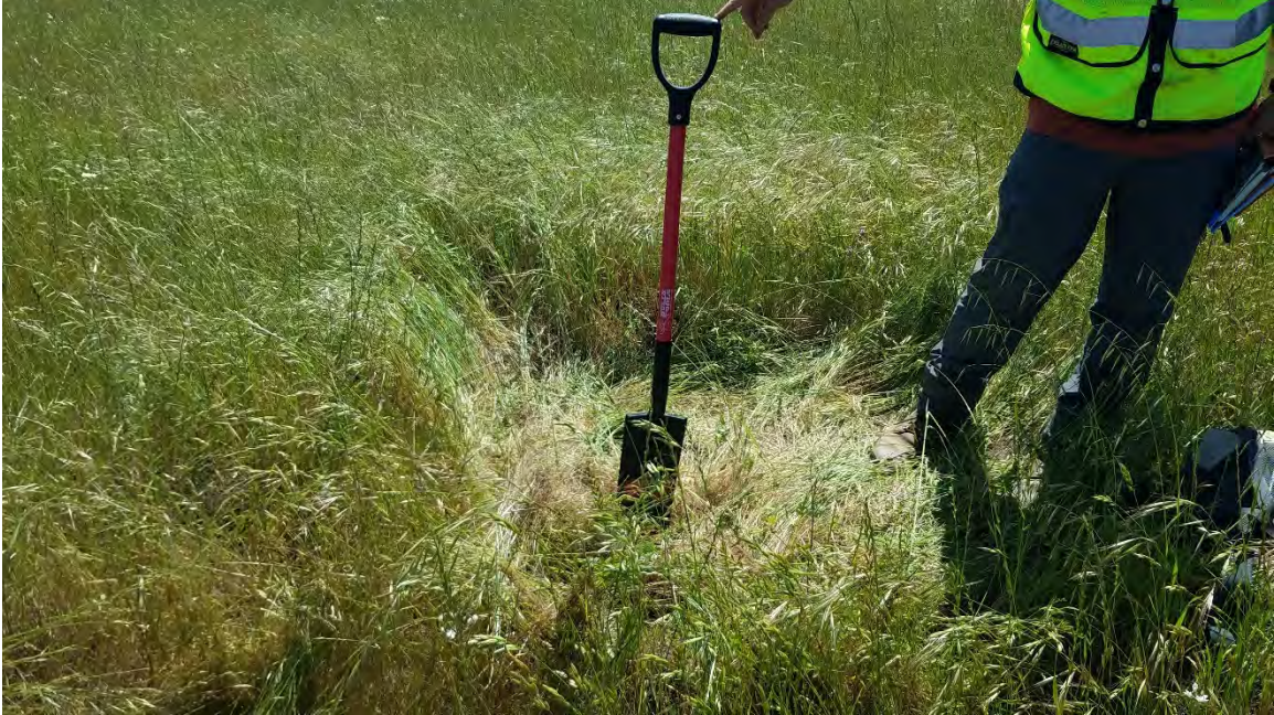
Arterial Roads Project. 170242
