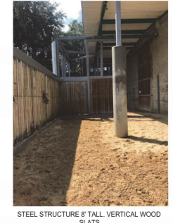
STEEL STRUCTURE 8' TALL VERTICAL WOOD SLATS
