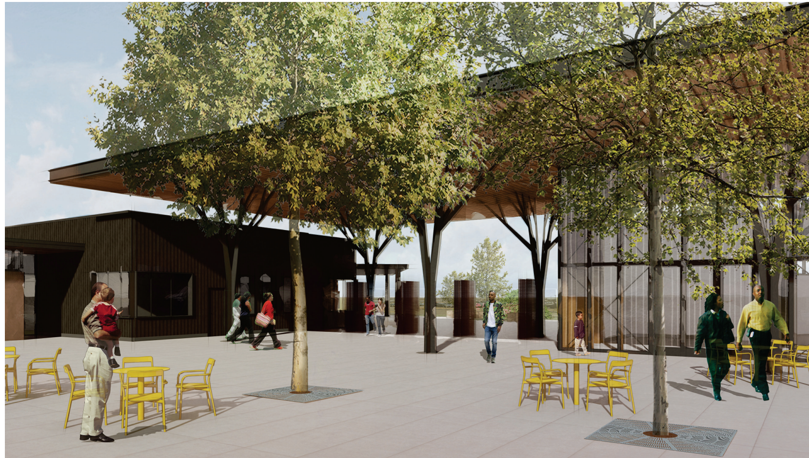
② CANOPY - STEEL PLATE BRANCHING TREE COLUMN
